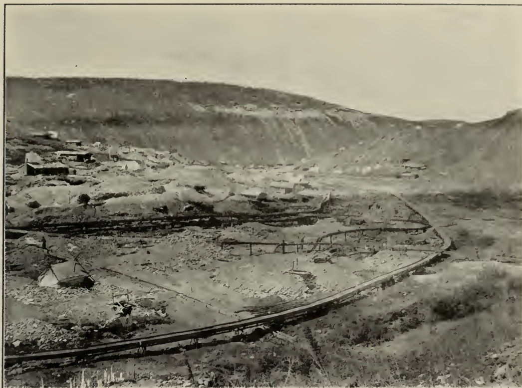
THE HIGHER WHITE LINE IN THE BACKGROUND SHOWS THE BENCH GRAVELS OF GOLD HILL. THE CREEK TO THE LEFT IS ELDORADO. IN THE FOREGROUND ARE THE CREEK CLAIMS OF BONANZA. $20,000,000 WERE PRODUCED FROM THE AREA SHOWN.
